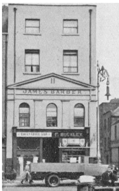
11 Aungier Street, now demolished. Photograph, T. S. Veitch, The Story of the Brethren Movement [1925].
